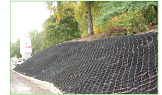
SLOPE EROSION CONTROL & SOIL RETENTION
