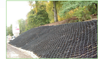
SLOPE EROSION CONTROL & SOIL RETENTION
